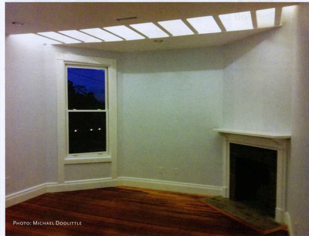
Ceiling framing is revealed by selective demolition to become a lighting-diffuser. In the same space, trim and fireplace are restored.
