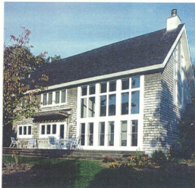
Plenty of windows on the western wall. Combining stock sizes of windows and doors in different patterns creates a custom look on a limited budget. Photo taken at E on floor plan.
