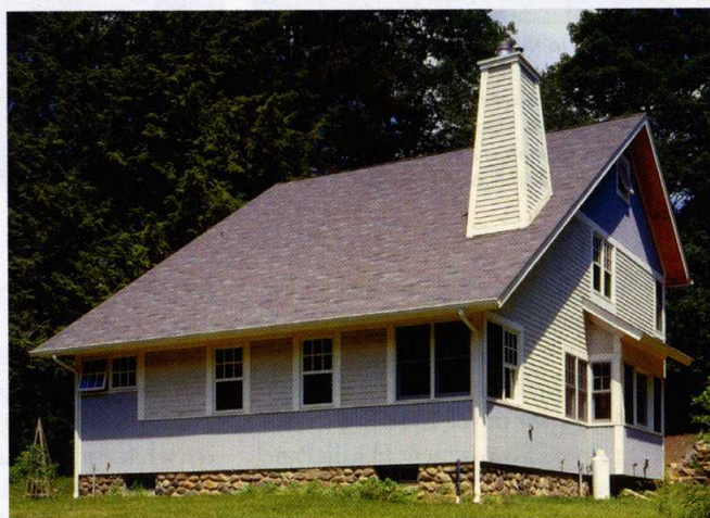
Modest budgets demand straightforward shapes and spaces. Part of an architect's job is to design a house that can be built on budget. For these cost-cutting clients, that meant simple framing (a basic roof shape) and simple materials (clapboards, T-111 siding, and asphalt roof shingles).
