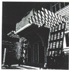
A cantilevered porch overlooks the marsh. Two large brackets and a large beam support a cantilevered porch off the master bedroom. Trellises with contoured tails flank the porch. Photo taken at G on floor plan.
