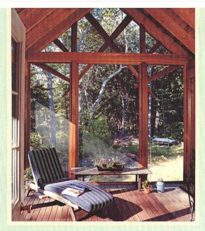
THE WALLS OF A SCREEN PORCH don't just keep the bugs out, they can also work as art. Here, simple trim pieces are cut to botanical shapes and applied to the outside face of the framing.
