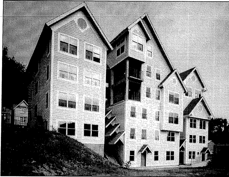
Figure 1-1 Cephass housing in downtown Yonkers, New York. Duo Dickinson, architect. Photo © Mick Hales.
