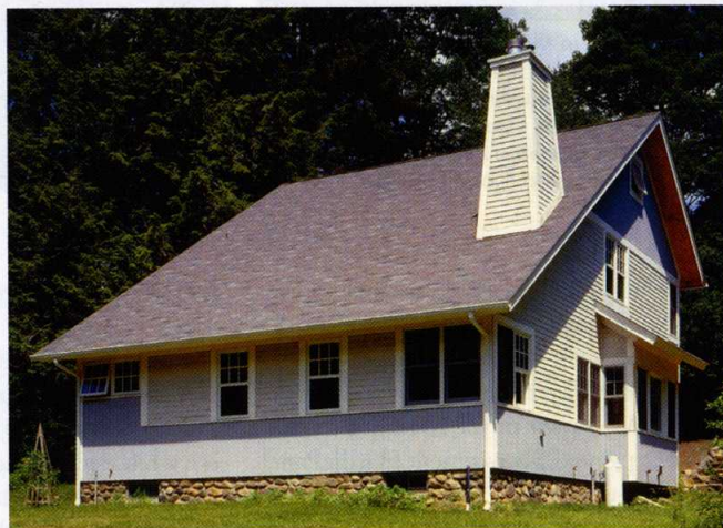
Modest budgets demand straightforward shapes and spaces. Part of an architect's job is to design a house that can be built on budget. For these cost-cutting clients, that meant simple framing (a basic roof shape) and simple materials (clapboards, T-111 siding, and asphalt roof shingles).
