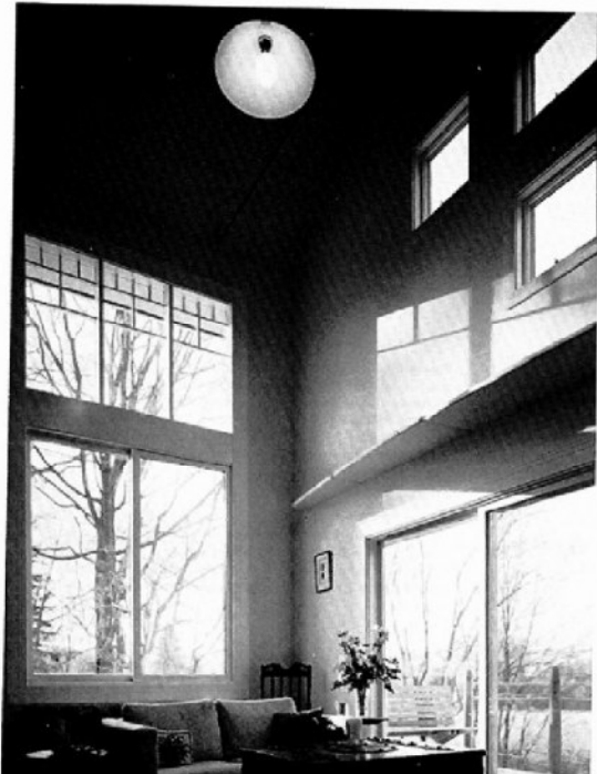
Figure 19 Living room, west. This ensemble of openings is the visual greeting the house provides once the occupant proceeds over the threshold. The westerly tall window is a duplicate of the window first apprehended upon access to the site. Made from a standard slide below and custom fixed unit above, the glazing division mimics the tree form opposite it, while the window's shape captures both the intense sunsets and the tree's ascendancy. The horizontal slider affords an uninterrupted sweep of the salt-marsh view. The cluster of square clerestory windows above (which forms a cruciform when fully depicted) is a centered array providing both ambient light and ventilation. The vertical, horizontal, and centered fenestration provide a minor-league compendium of the orientations possible in any glazing system. Note the tie-rod orientation to the west window, which in turn is oriented to the fireplace opposite, creating a minor subaxis.
