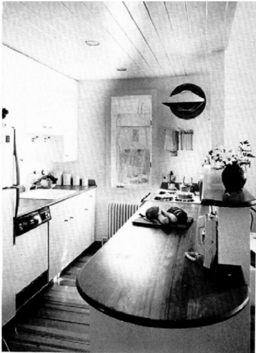
Figure 18 Kitchen and entry view. Simple, inexpensive cabinets are opposed to create a galley kitchen. The axis created between the cabinets centers upon the front door and orients the radiator and window as well. Teak counters and a custom range hood enliven the entry vantage.
