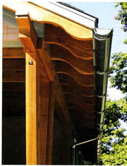
The eaves that CK Architects added use natural wood — in this case Douglas cut to a decorative outline — and raw aluminum gutters to counterpoint the painted trim and siding.
