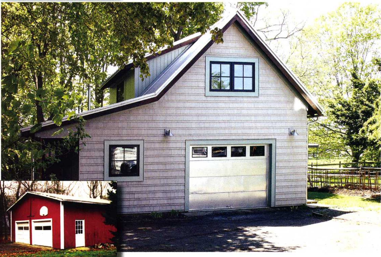
Before (inset) and after views of both the house and the faux barn garage (below), which became virtually a new building, with studio above and shop on the ground floor.
